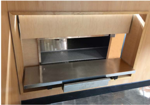
When the door is open, the conveyor stops moving for easy loading.
